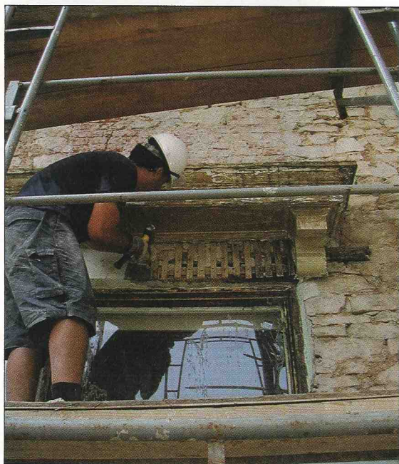
Above: Stucco was removed carefully from this window hood. Right: Today this same window is picture-perfect after its final coat of stucco.
