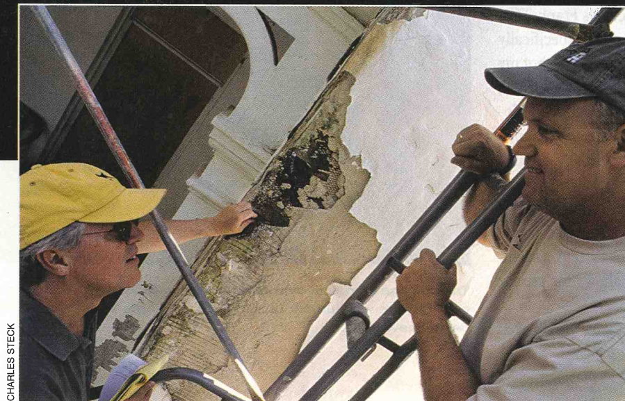
Left: Project architect Doug Gilpin and Rich Baker of Tidewater Preservation discuss the extent of the failed stucco at Morven Park.
